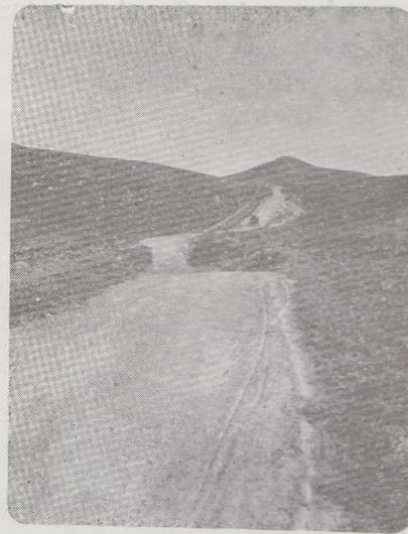
FROM THE STATION AT NOTTINGHAM ROAD TO THE BUNGALOW.
