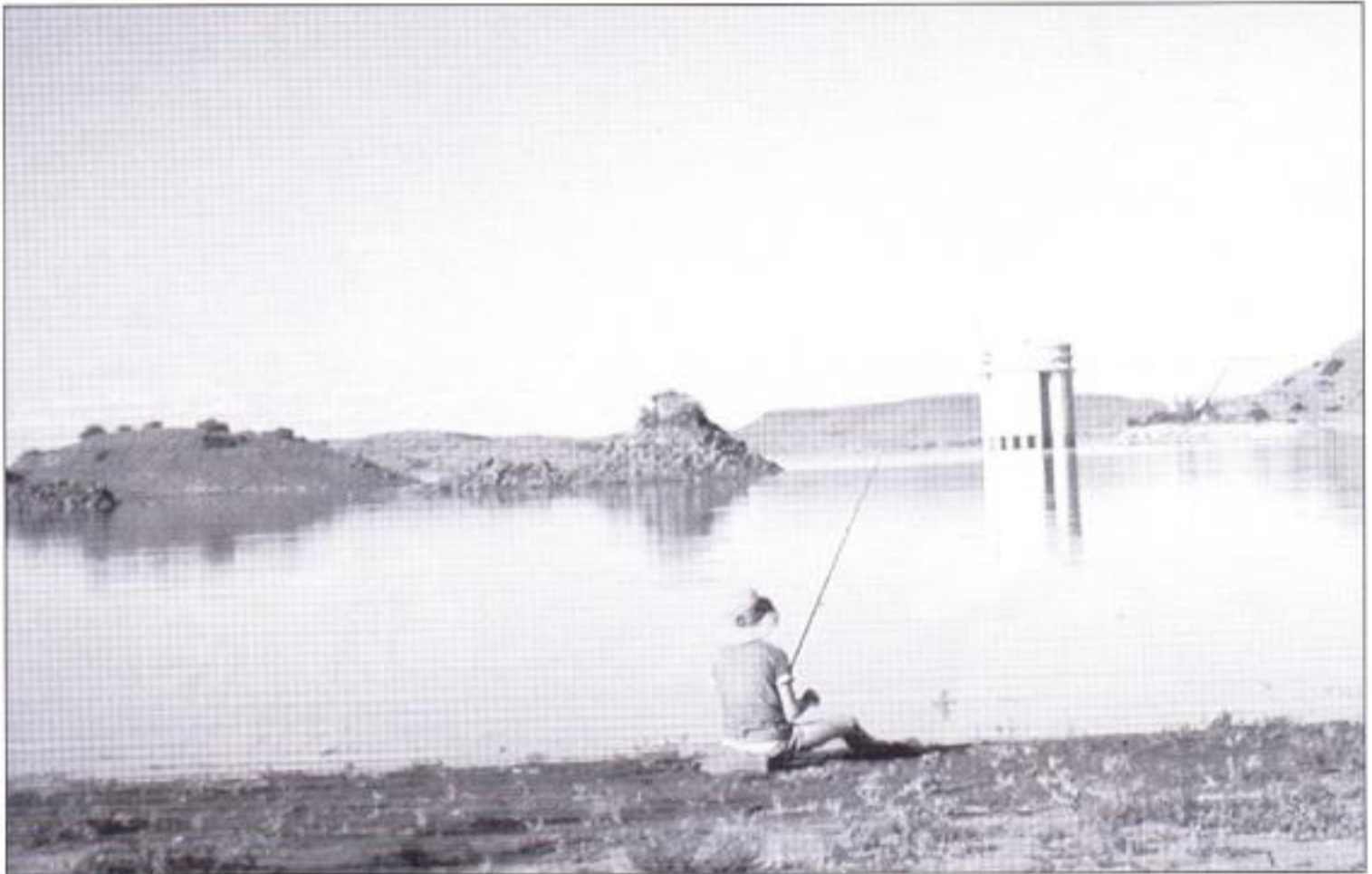
The Orange Fish tunnel inlet situated in the Gariiep Dam on the Orange River, a conduit for introducing barbel into the Fish River.
